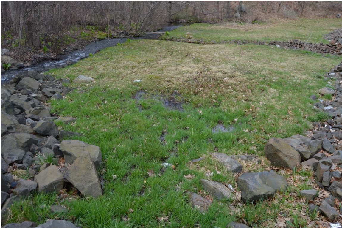
Photo 21c – Saturated ground between the toe of the left downstream embankment and the downstream channel.
