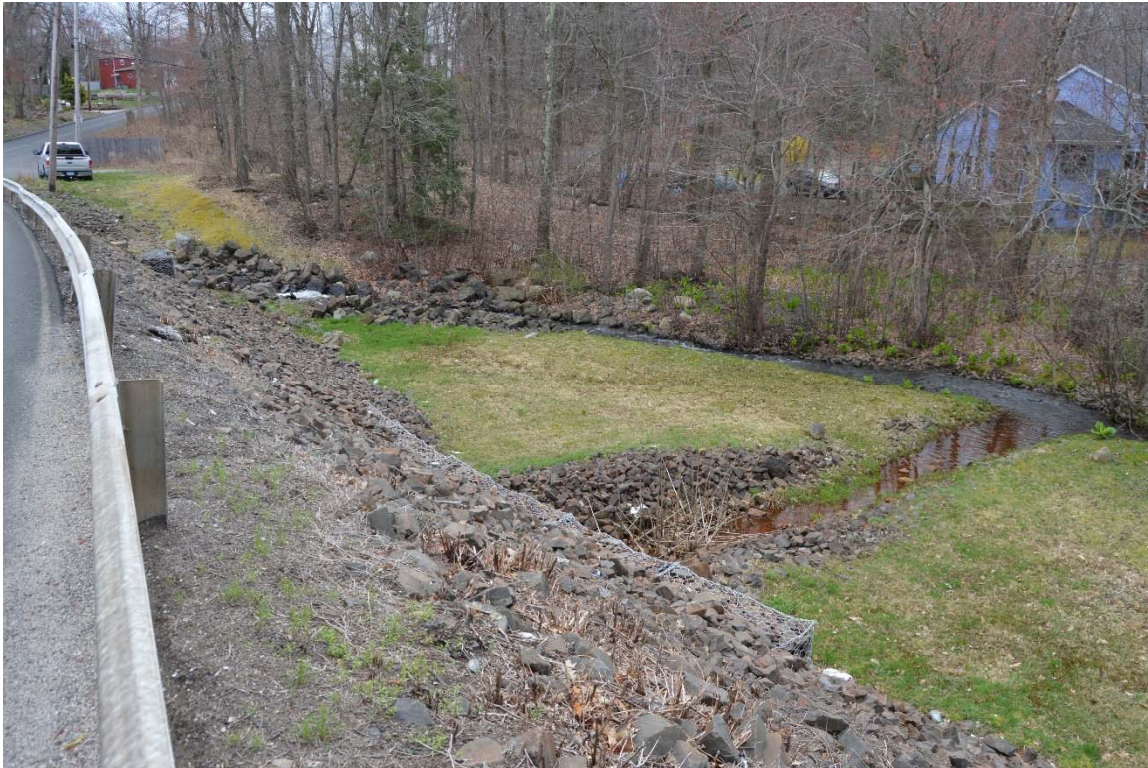
Photo 7a – An overview of the downstream face and toe area, taken from the right side of the embankment. The discharge channel for the low level outlet is at the right-center of the photo.
