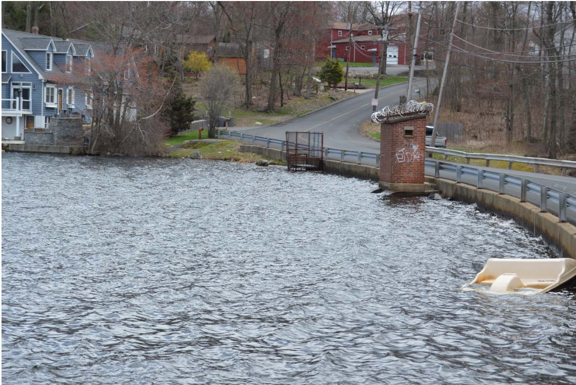
Photo 1a – Cedar Lake Dam, as seen from the right upstream abutment.
