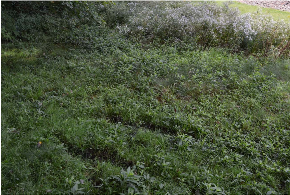
Photo 21o – Rutting from vehicular tracks in the downstream base area, probably caused by mowing equipment being driven through a wet area. Such sections may have to be mowed with a hand-push mower or weed whacked.
