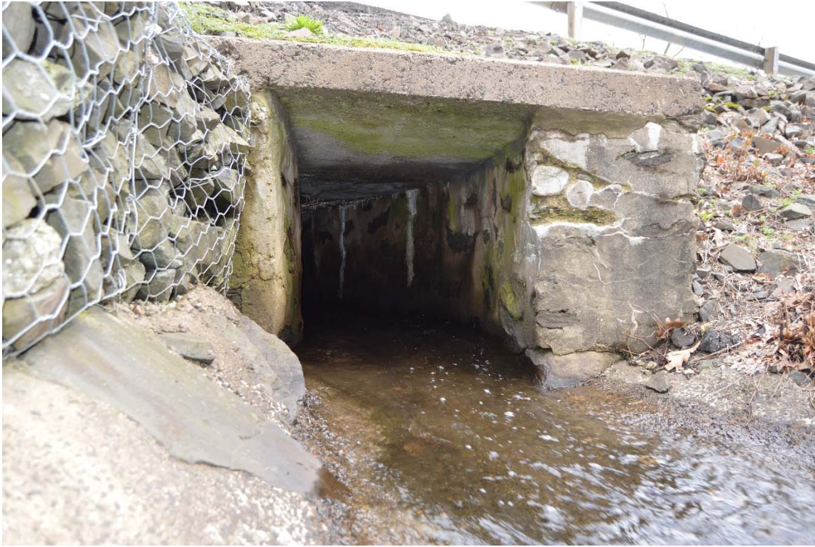
Photo 19c – The downstream end of the tunnel conveying the spillway discharge flow.
