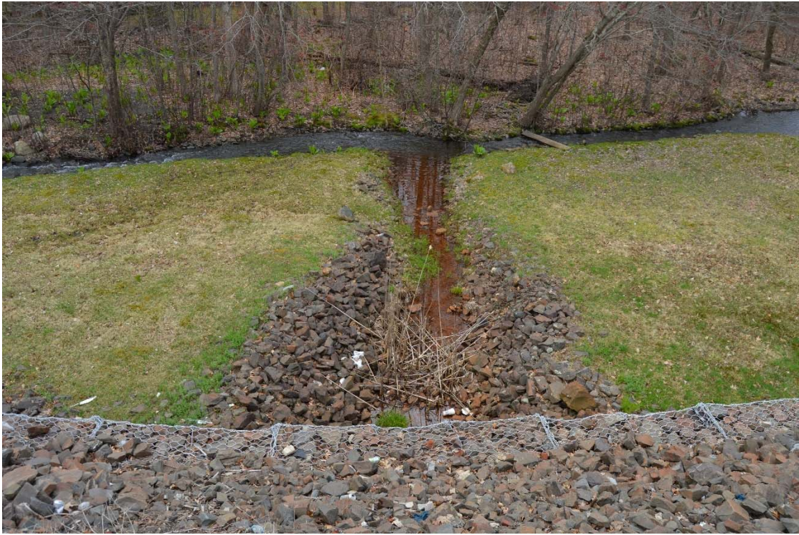
Photo 15c – The low level outlet discharge channel, from the pipe end to the junction of the channel with the main stream (Mad River) in the center background of the photo.
