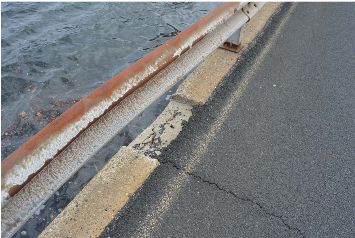
Photo 19h – A curb cut on the north (upstream side) of North Street, facilitating the discharge of flow runoff from the road into the impoundment on the north side of the road.
