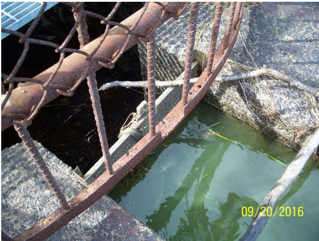
Photo 13b – The spillway weir, with weir boards in place, as seen through the protective fencing in 2016.
