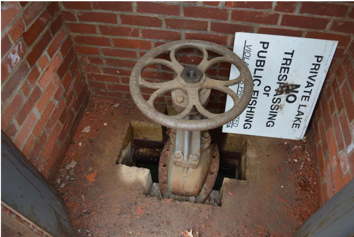
Photo 17a & 18a – The interior of the gatehouse and the operator for the sluice gate at the low level outlet.
