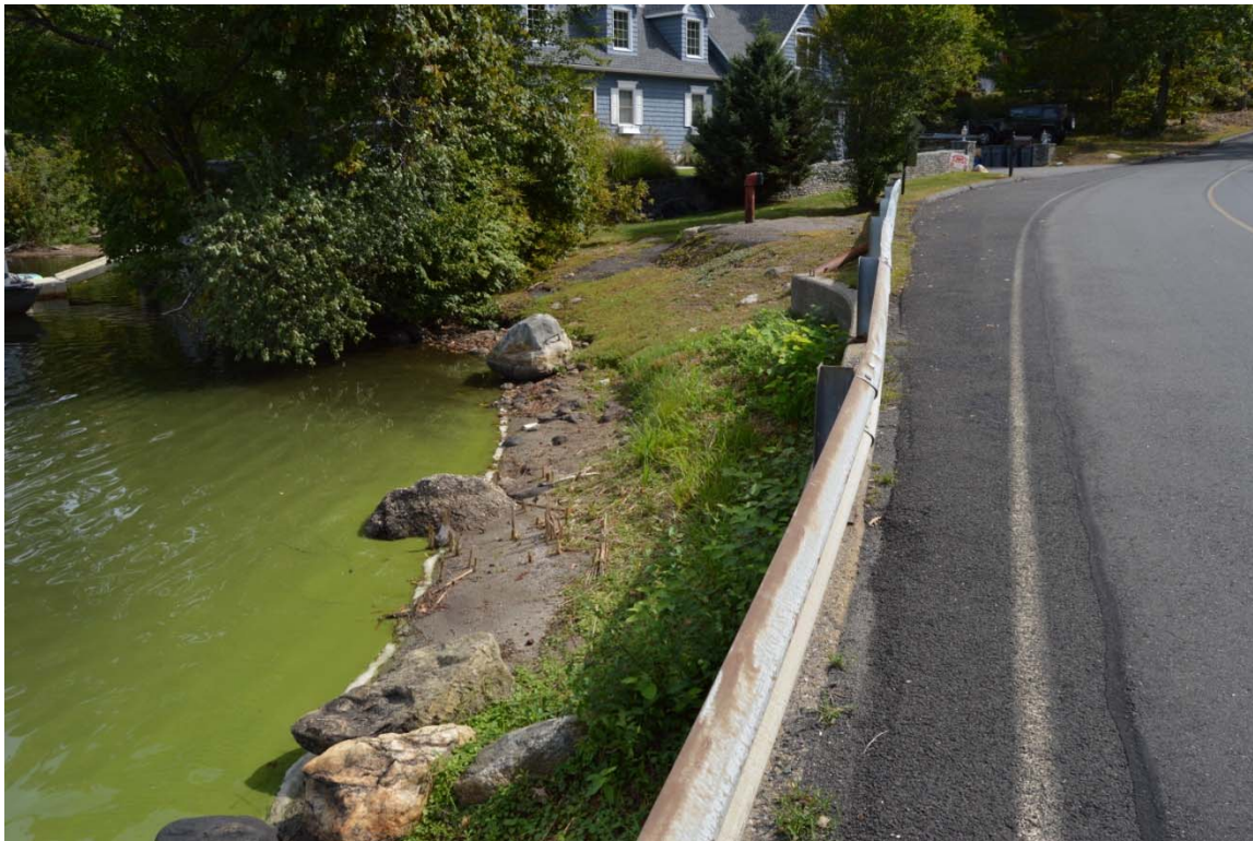
Photo 4e – A view of the left side upstream embankment area, as taken from North Street during a low water level period in 2016.
