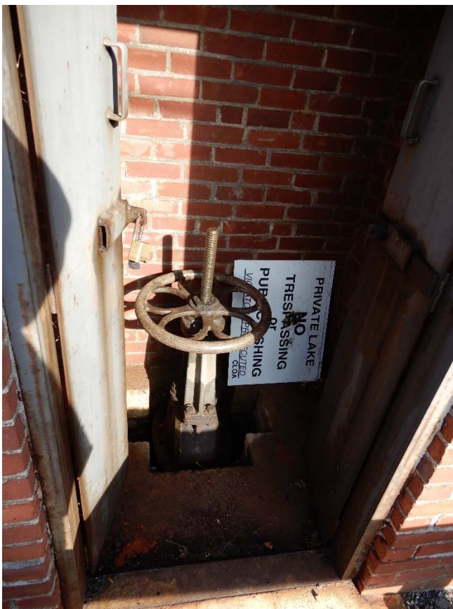
Photo 17a & 18a – The interior of the gatehouse and the operator for the sluice gate at the low level outlet.
