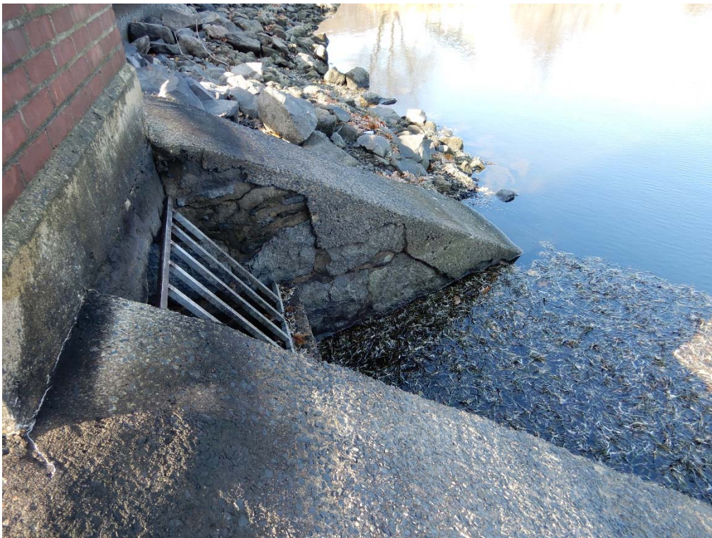
Photo 21p – The stubby right side training wall at the base of the gatehouse and low level intake area. The concrete cap over the stone masonry and concrete surfaces should be inspected during annual drawdowns for any potential defects.
