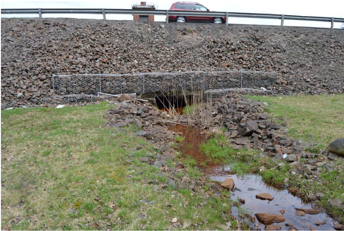
Photo 19a – The downstream end of the low level outlet discharge structure.
