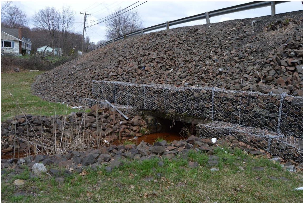
Photo 14b – The same discharge area as seen in the prior photo, taken from its left side. Although minor vegetative growth is visible in the channel, it is typically cleaned out on a seasonal basis.
