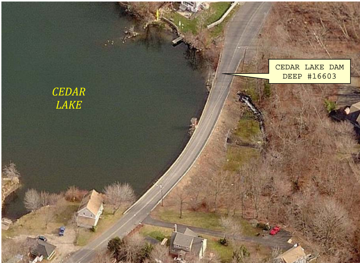
Another aerial view of Cedar Lake Dam, looking eastward from the right side of the dam. (Source: Bing Maps)
