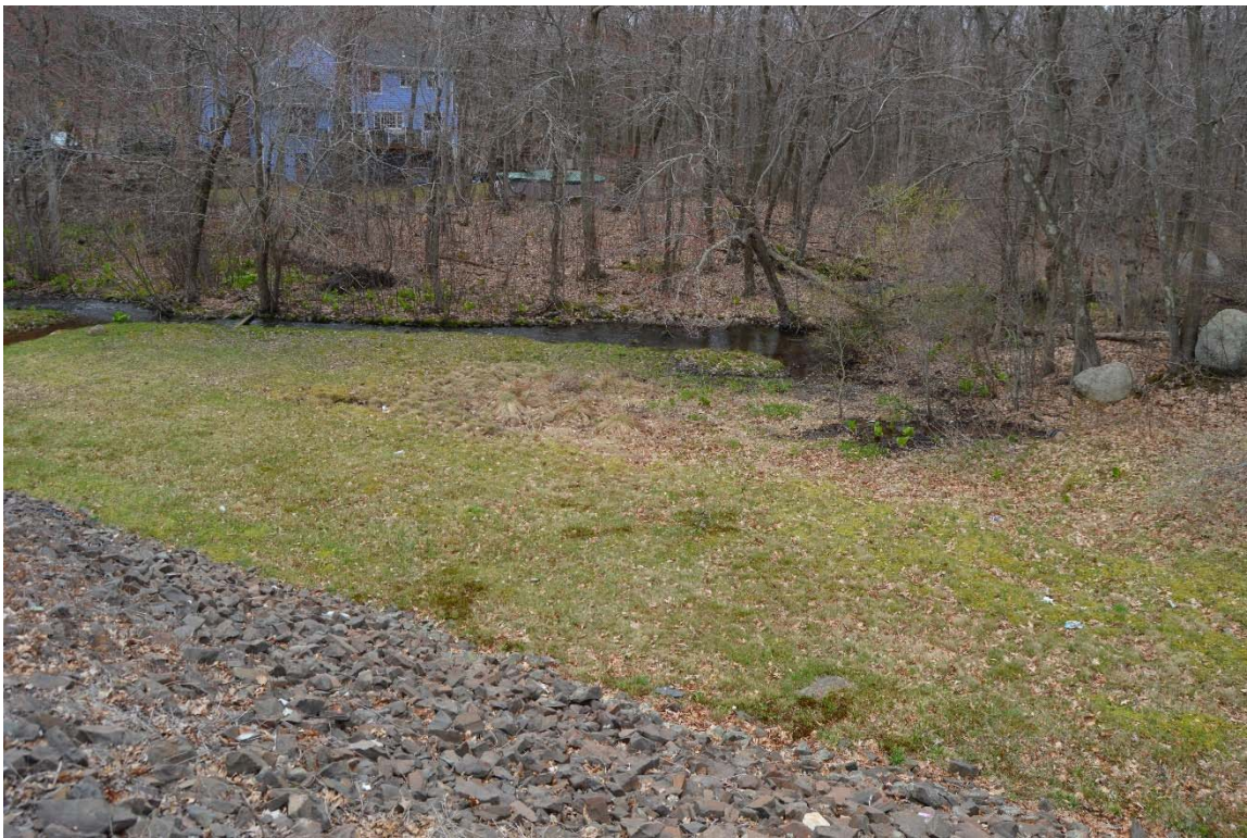
Photo 15f – The lower reaches of the downstream channel, continuing southward as the Mad River.
