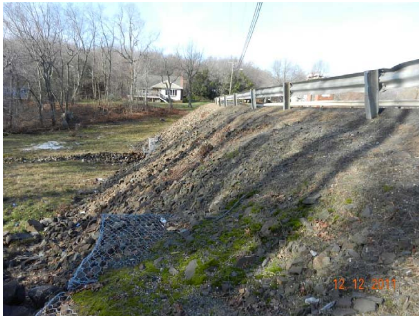
Photo 10: Downstream side of Dam/Road Embankment
