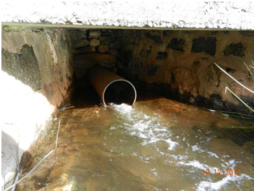
Photo 14: Outflow of Low Flow Outlet
