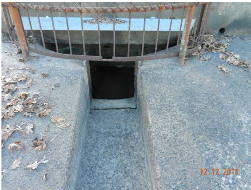
Photo 4: Horizontal & Semicircular Weir of High Flow Outlet
