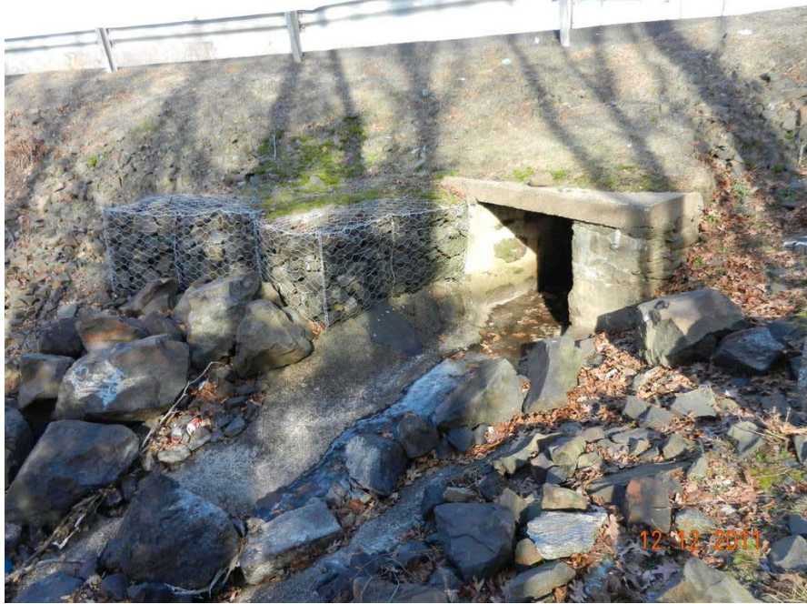
Photo 11: Outflow of Box Culvert (High Flow Outlet)
