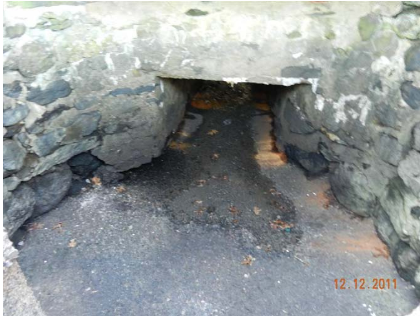
Photo 5: Box Culvert of High Flow Outlet
