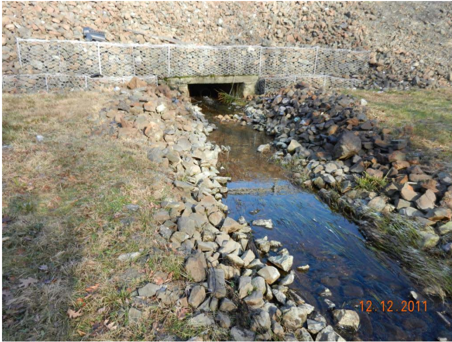
Photo 13: Outflow of Low Flow Outlet
