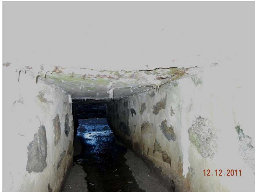
Photo 12: Box Culvert of High Flow Outlet
