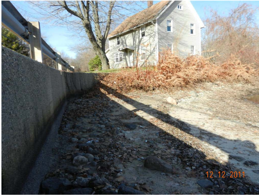
Photo 9: Retaining Wall on upstream side of Dam
