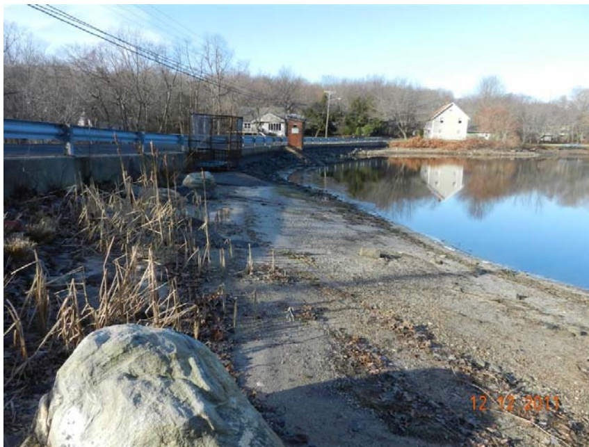
Photo 2: Upstream side of Cedar Lake Dam
