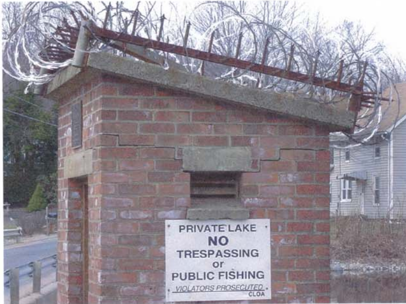
Photo 21 - The left side of the gatehouse, with a crack emanating from the top of the right window corner. While not a serious problem at this time, the crack should be repaired to avoid more serious displacement with continued exposure to the elements.
