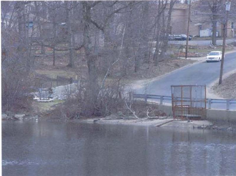
Photo 17 - The primary spillway near the left end of the dam. Note here the growth of woody vegetation and a tree within 25 feet of the end of the dam, both of which should be removed.
