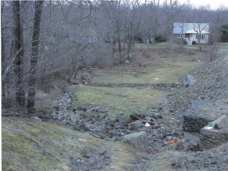
Photo 1 - An overview of the downstream side of the dam embankment. Note the growth of small trees at the right center of the photo, debris and displaced riprap at the discharge opening of the spillway channel and the wet area at the right downstream side of the dam.
