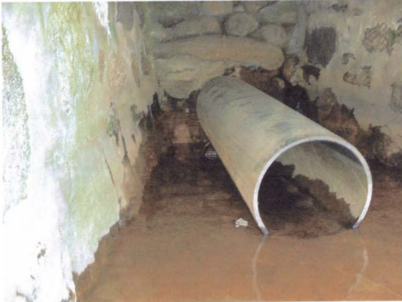
Photo 9 - Seepage is also present along the wall on the right side of the low level outlet pipe. Again, this flow should be monitored for any changes, but no further action is required at this time.
