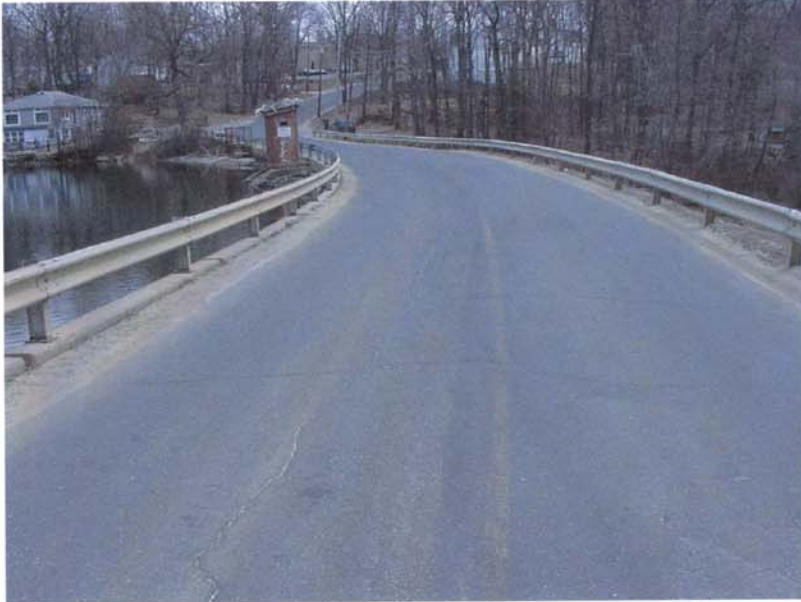
Photo 15 - The top of the dam consists of the Town road, which in general appears slopes toward the upstream side of the dam. Although there are leak-offs through the concrete wall crest, the buildup of sand sediment indicates areas of ponding which may lead to infiltration into the embankment through cracks in the roadway.
