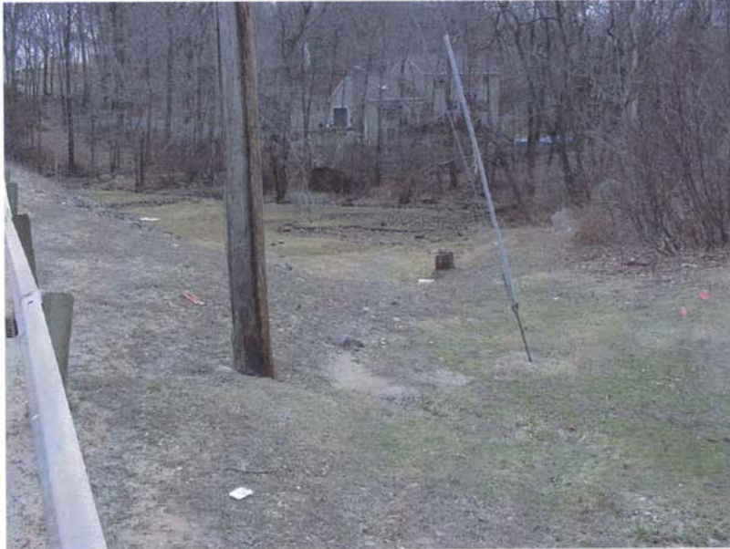
Photo 13 - The right end of the downstream embankment; the drainage pipe mentioned in the previous photos runs adjacent to the pole guy wire with the discharge at the base of the embankment near the center of the photo. Note the lack of vegetation along the embankment crest and sediment near the pole from apparent surface runoff at the road.
