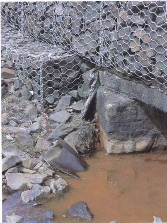
Photo 9 - Seepage is also present along the wall on the right side of the low level outlet pipe. Again, this flow should be monitored for any changes, but no further action is required at this time.
