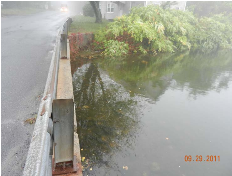
Photo 8 – A view toward the right upstream end of the dam showing thick vegetation along the upstream wall section.
